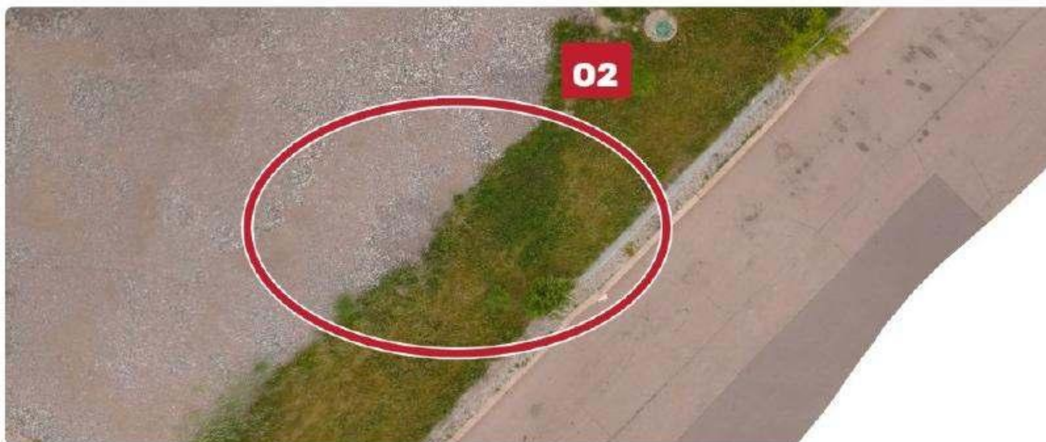
02.1 – SP3 toe beside the grassed boulevard, with no perimeter control visible.
