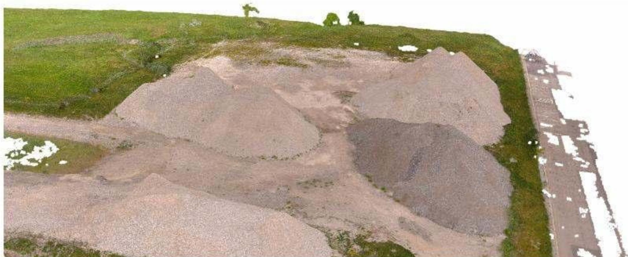
Figure 5.2 · Stockpile area, close oblique view
