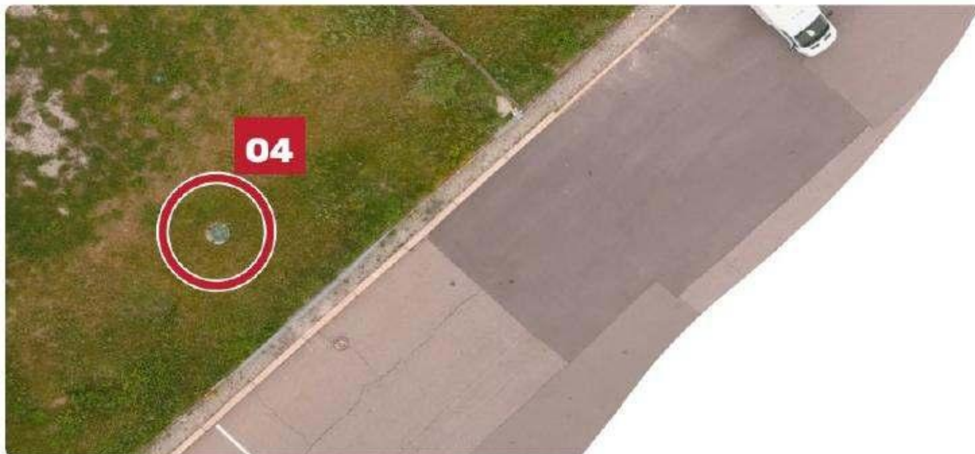
04.2 – Access cover in the grassed area near the parking frontage.
