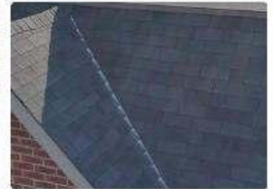
Photo 18 Front mansard slope & dormers
