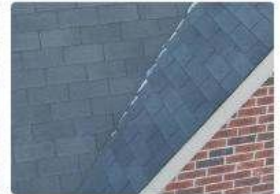
Photo 11 Front mansard slope & dormers
