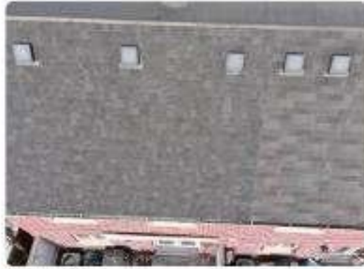
Photo 81 Rear mansard slope & transition
