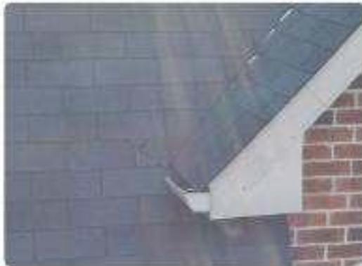
Photo 8 Front mansard slope & dormers
