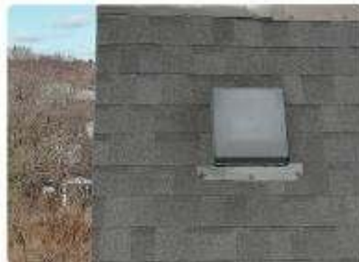
Photo 117 Rear slope close-ups
