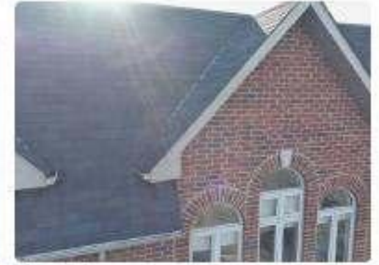
Photo 7 Front mansard slope & dormers
