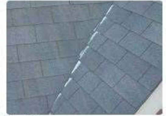
Photo 31 Front mansard slope & dormers
