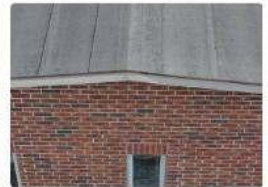
Photo 45 Upper roof & end wall overview
