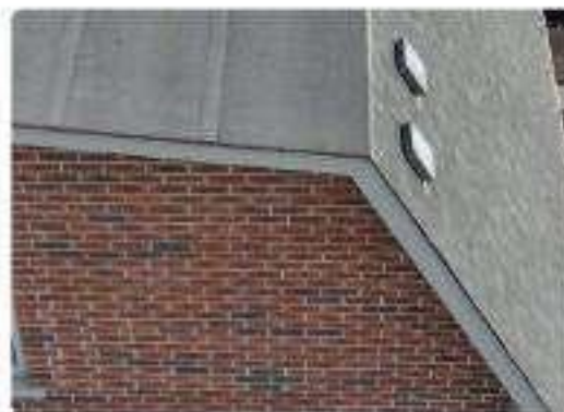
Photo 47 Upper roof & end wall overview
