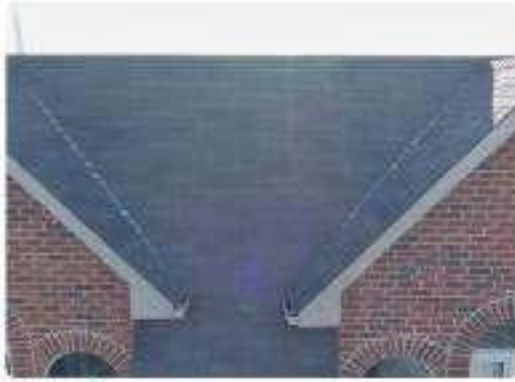
Photo 1 Front mansard slope & dormers
