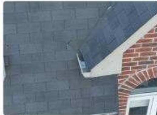
Photo 13 Front mansard slope & dormers
