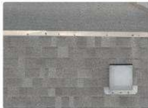
Photo 64 Rear mansard slope & transition
