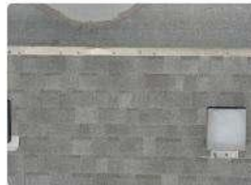
Photo 65 Rear mansard slope & transition
