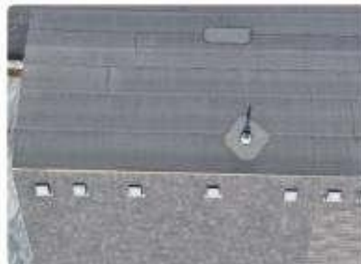
Photo 76 Rear mansard slope & transition
