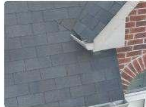
Photo 34 Front mansard slope & dormers
