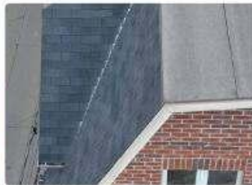
Photo 43 Upper roof & end wall overview
