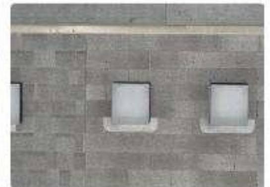
Photo 66 Rear mansard slope & transition
