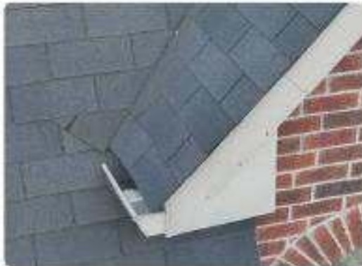
Photo 32 Front mansard slope & dormers
