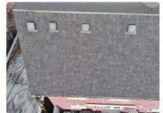
Photo 80 Rear mansard slope & transition
