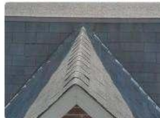
Photo 26 Front mansard slope & dormers
