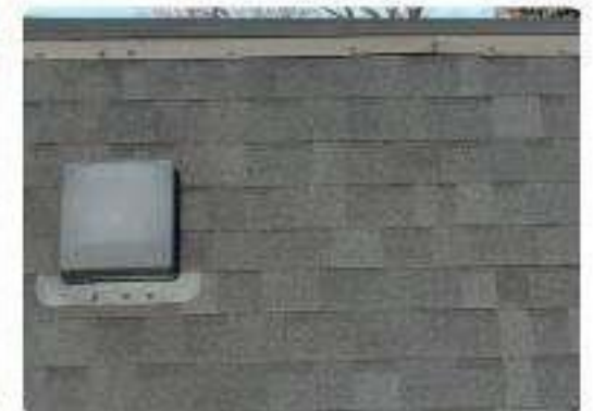
Photo 119 Rear slope close-ups
