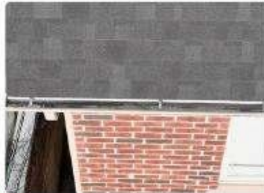
Photo 86 Rear eave & eavestroughs
