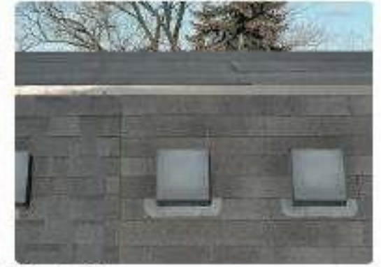
Photo 123 Rear slope close-ups
