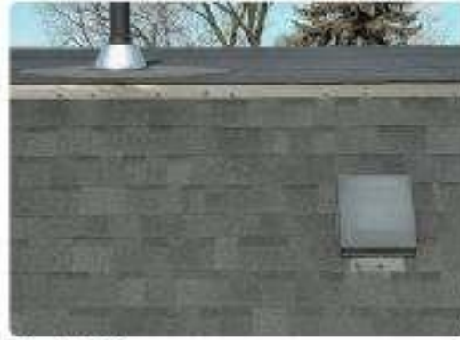
Photo 121 Rear slope close-ups
