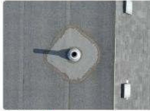
Photo 56 · F5 Low-slope membrane
