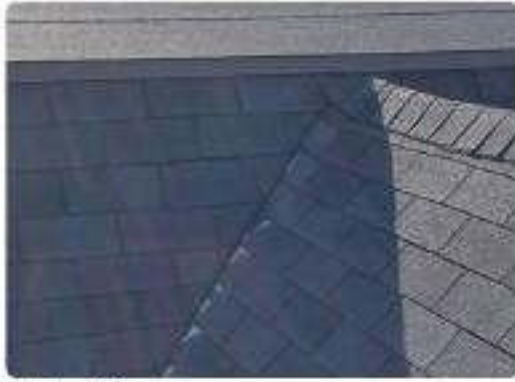
Photo 28 Front mansard slope & dormers
