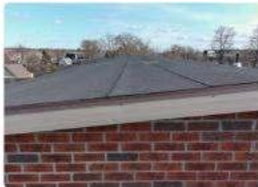
Photo 101 End wall, rake & perimeter
