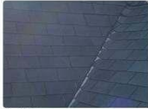
Photo 29 Front mansard slope & dormers
