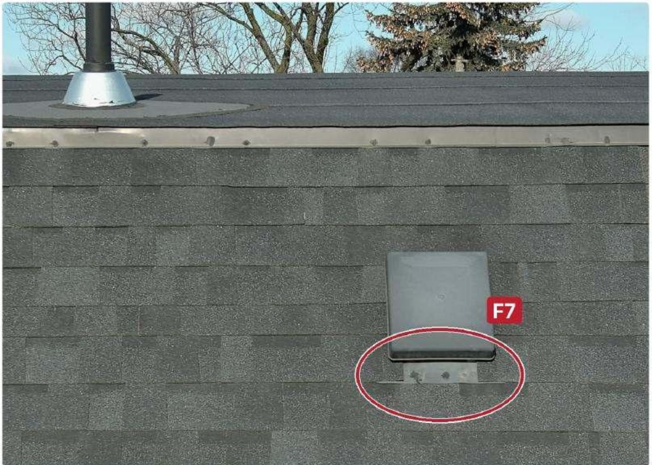
F7.1 – Face-fastened lower flange on a box vent.
