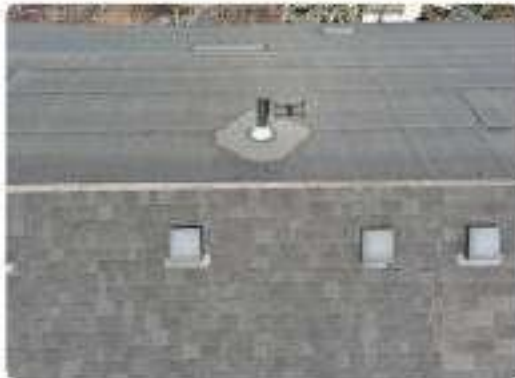
Photo 59 Rear mansard slope & transition
