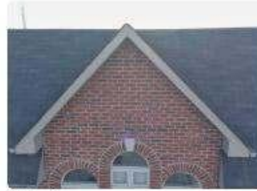
Photo 3 Front mansard slope & dormers
