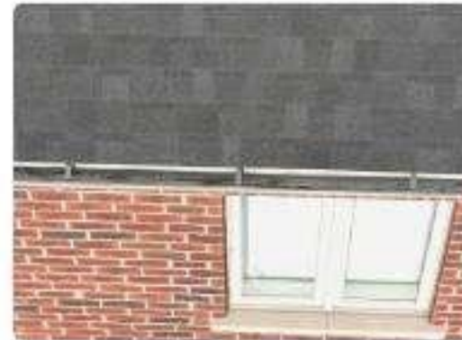
Photo 87 Rear eave & eavestroughs
