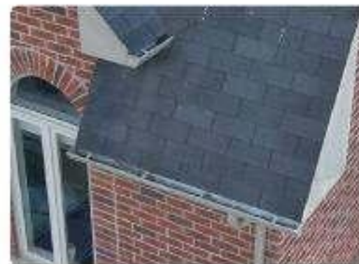
Photo 21 Front mansard slope & dormers
