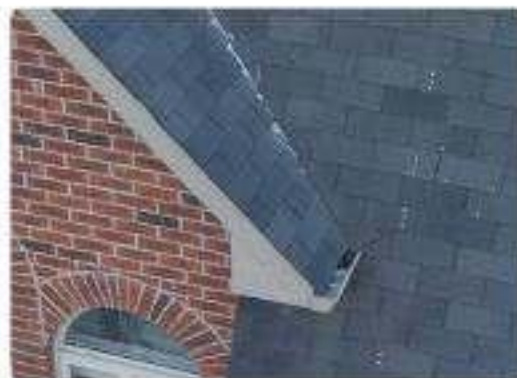
Photo 20 · F3 Front mansard slope & dormers
