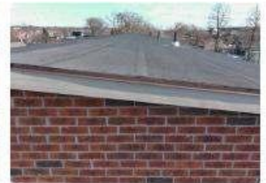
Photo 104 End wall, rake & perimeter
