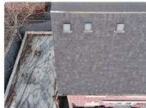
Photo 79 Rear mansard slope & transition
