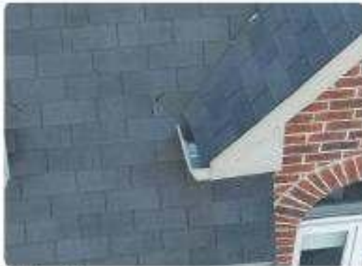
Photo 12 Front mansard slope & dormers
