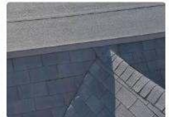
Photo 27 Front mansard slope & dormers
