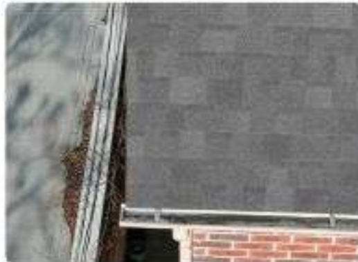
Photo 85 Rear eave & eavestroughs
