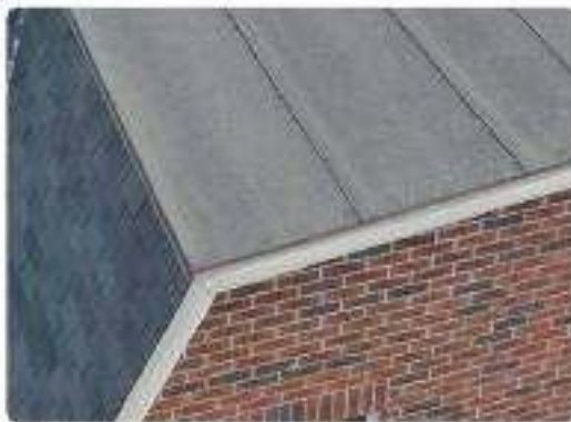
Photo 42 Upper roof & end wall overview
