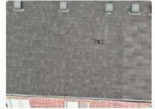
Photo 84 Rear mansard slope & transition
