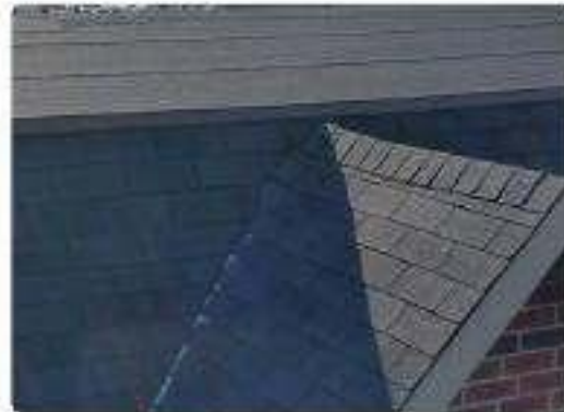
Photo 9 · F2 Front mansard slope & dormers
