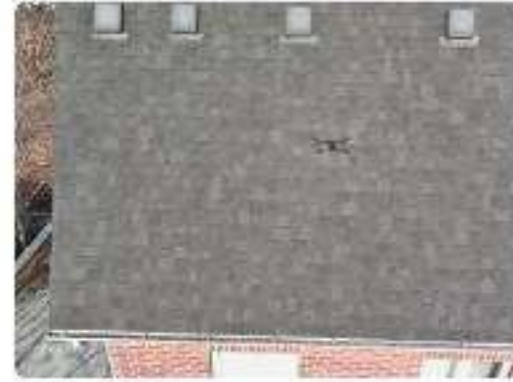
Photo 83 Rear mansard slope & transition
