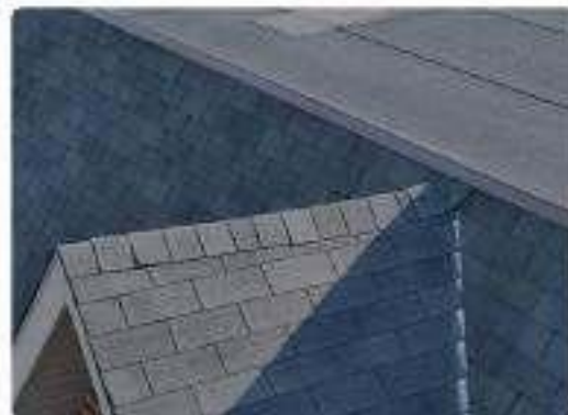
Photo 25 · F2 Front mansard slope & dormers
