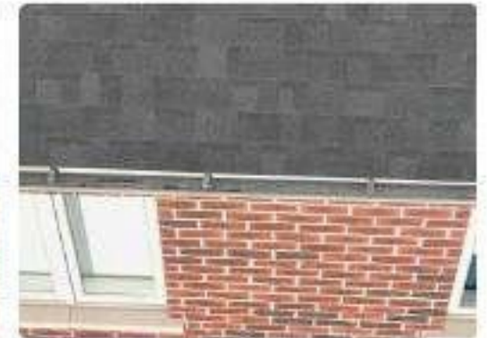
Photo 88 · F6 Rear eave & eavestroughs
