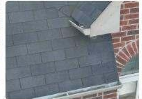
Photo 35 Front mansard slope & dormers
