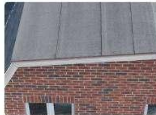
Photo 44 Upper roof & end wall overview
