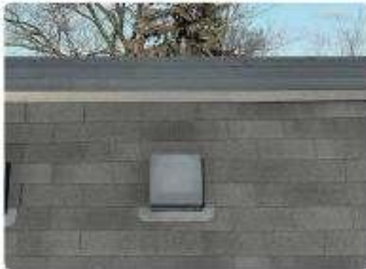
Photo 124 Rear slope close-ups
