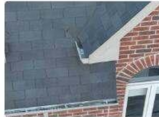
Photo 14 · F6 Front mansard slope & dormers
