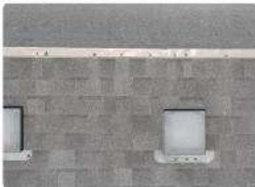
Photo 63 Rear mansard slope & transition
