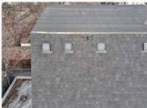
Photo 73 Rear mansard slope & transition
