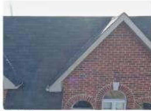
Photo 2 Front mansard slope & dormers
