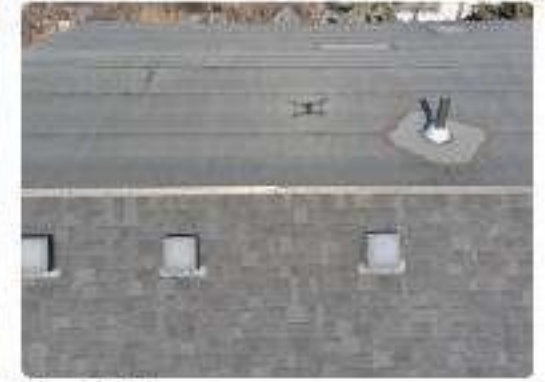
Photo 58 Rear mansard slope & transition
