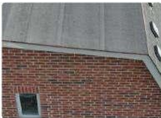
Photo 46 Upper roof & end wall overview
