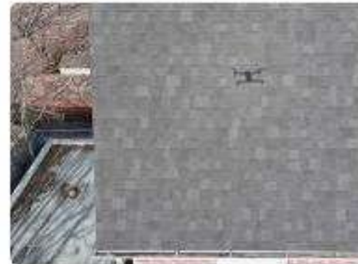
Photo 126 Rear slope close-ups
