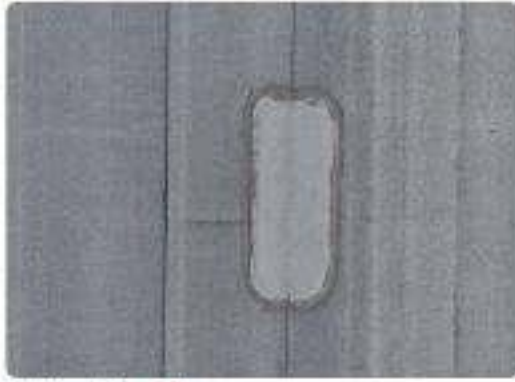
Photo 55 · F5 Low-slope membrane
