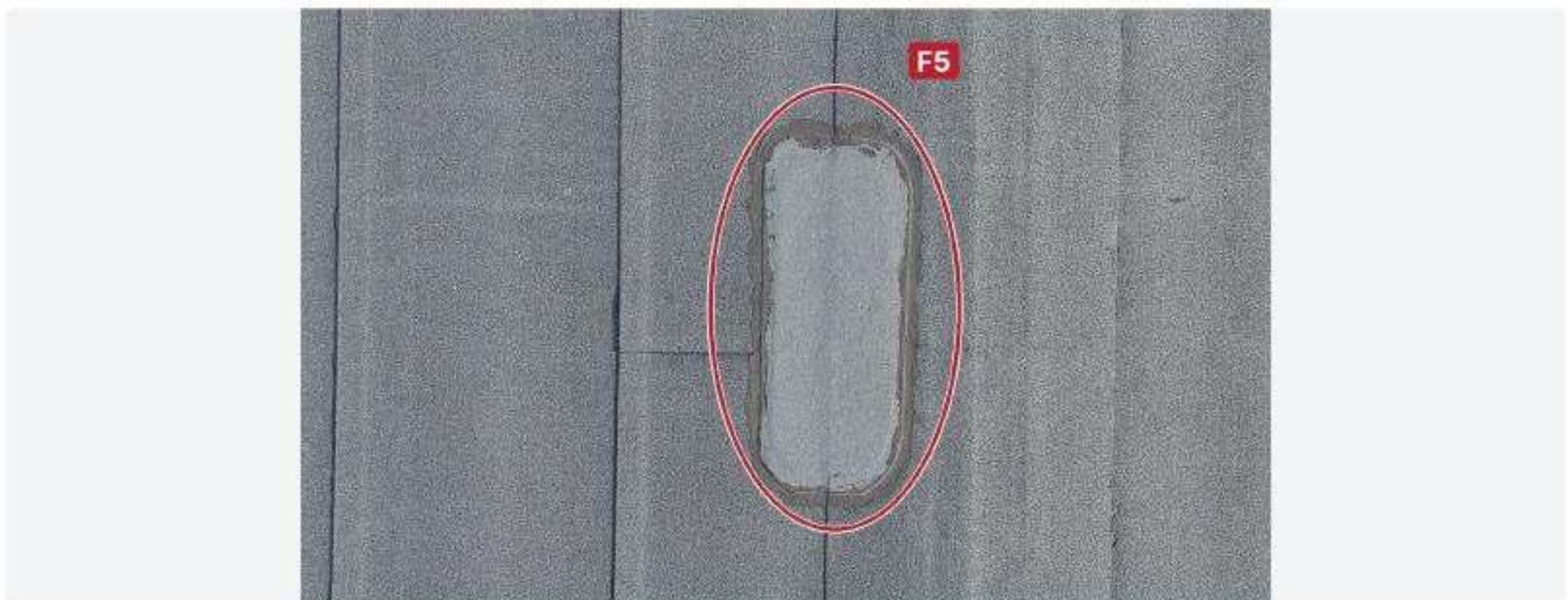
F5.2 – Rectangular target patch on the membrane.
