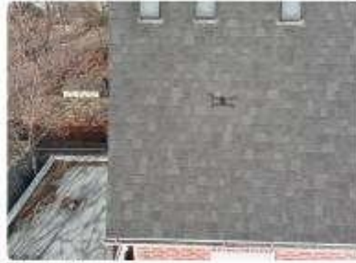
Photo 82 Rear mansard slope & transition
