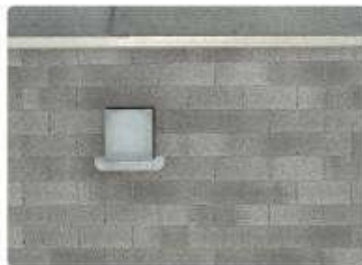
Photo 68 Rear mansard slope & transition
