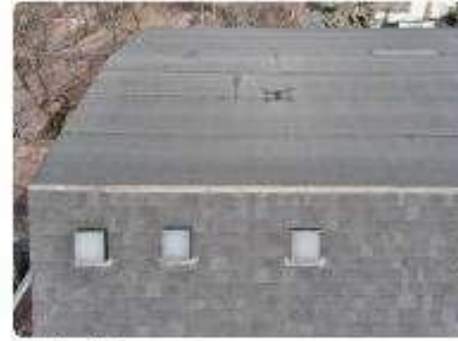
Photo 57 Rear mansard slope & transition
