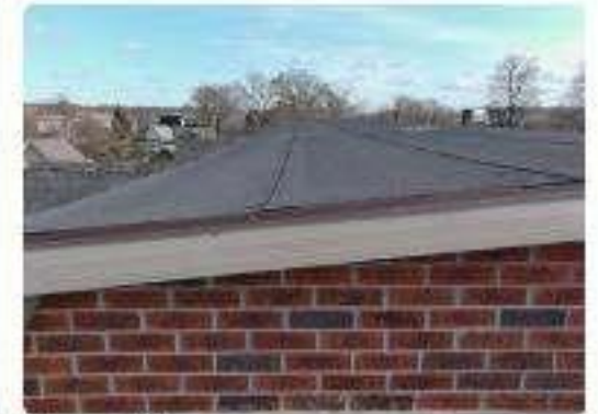
Photo 100 End wall, rake & perimeter
