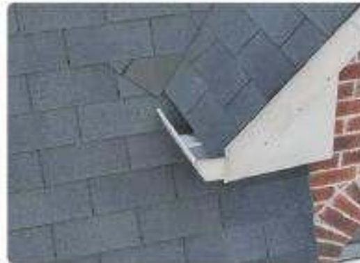
Photo 33 Front mansard slope & dormers
