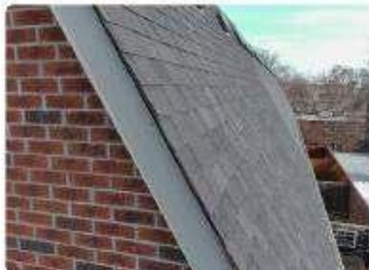
Photo 111 End wall, rake & perimeter
