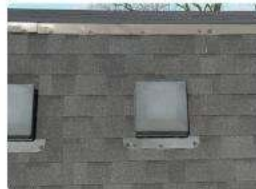
Photo 118 Rear slope close-ups
