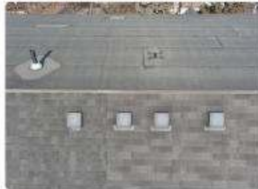
Photo 60 Rear mansard slope & transition
